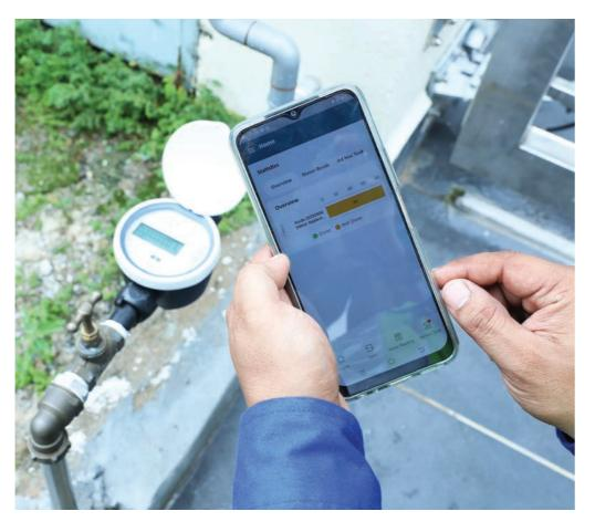
Air Selangor has embarked on a digital solution that empowers the Company and its customers through the smart water meter technology. The journey began in 2018 when Air Selangor conducted a pilot project to install 6,000 Automatic Meter Reading (AMR) devices in the Gombak, Kuala Lumpur and Petaling Jaya regions. From there, the project progressed to more advanced Ultrasonic Smart Meter (USM) technology with the approved installation of 50,000 USMs for 2023.
