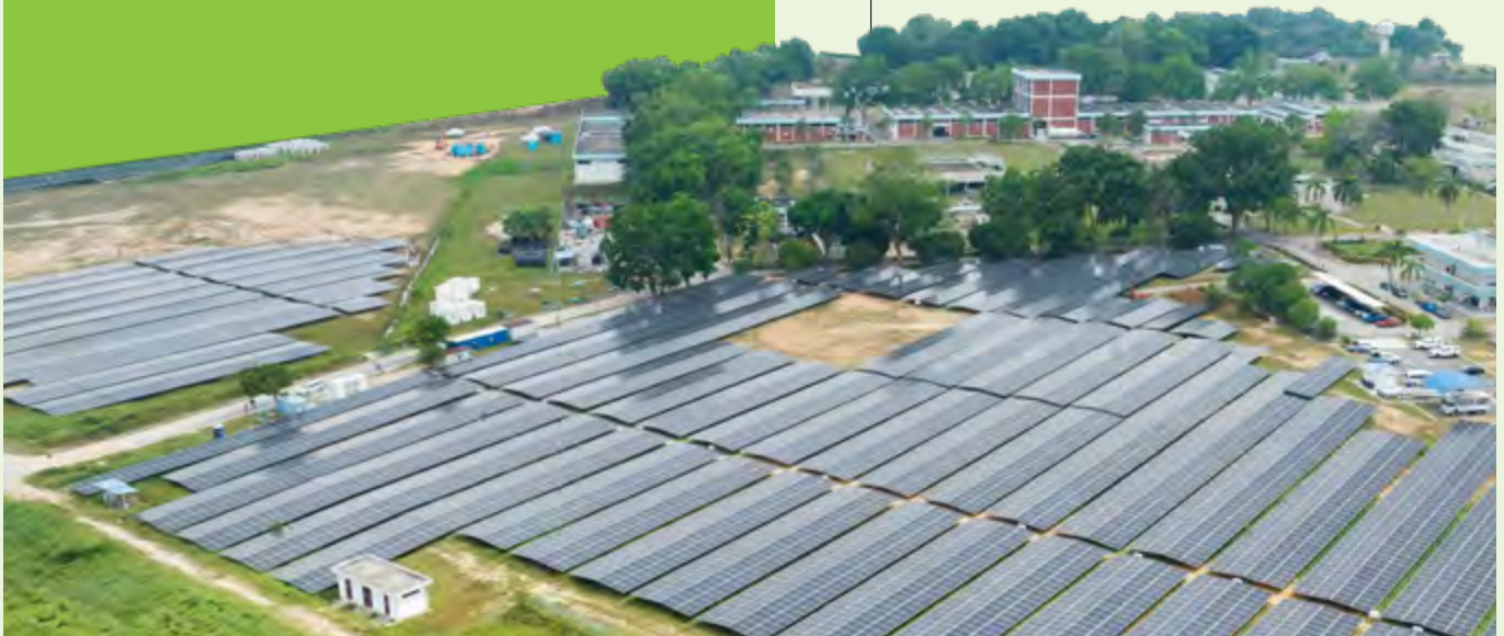
Solar Panels at Sungai Selangor Phase 2 (SSP2) Water Treatment Plant
