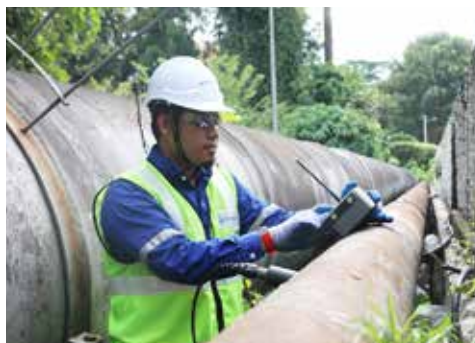
▶ Air Selangor's Leak Specialist (LS) and Leak Inspector (LI) teams detect pipe leak cases within the entire pipeline network using sounding equipment. To date, Air Selangor has a total of 54 LS and 133 LI personnel.
